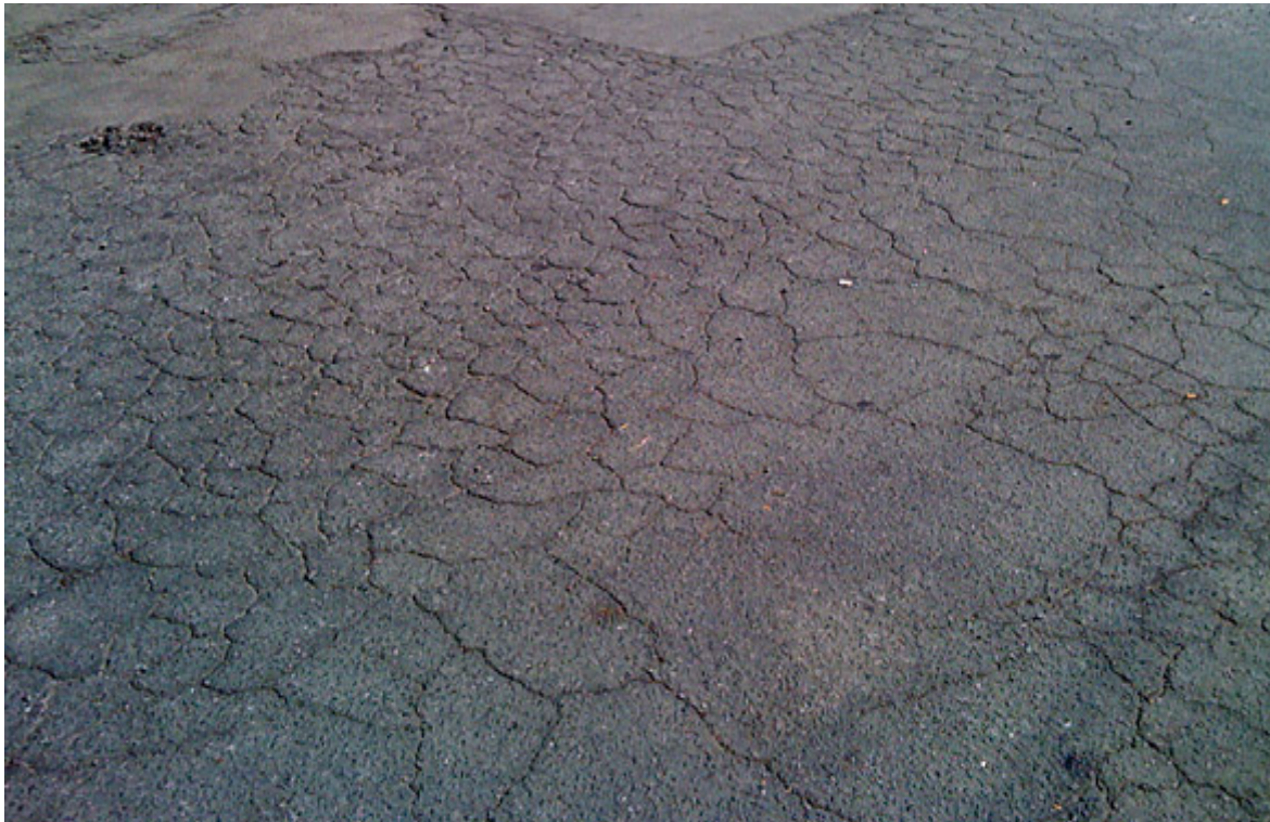
(1) Alligator Cracking
